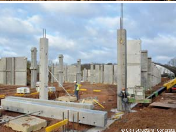
© CRH Structural Concrete
