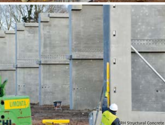
© CRH Structural Concrete
