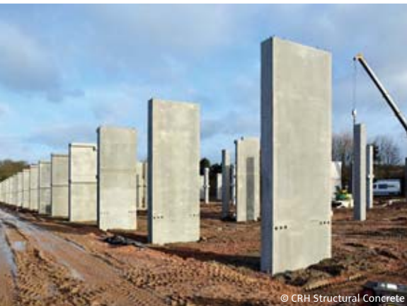
© CRH Structural Concrete
